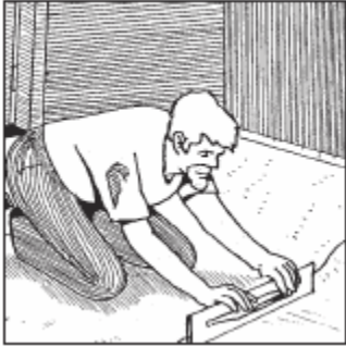
1. Level the sub-floor
